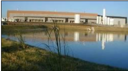
Rain Water Reuse Pond
